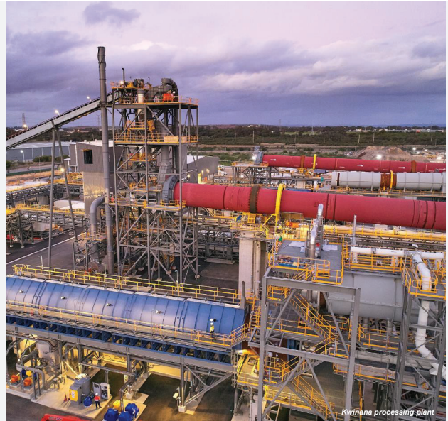
Kwinana processing plant
